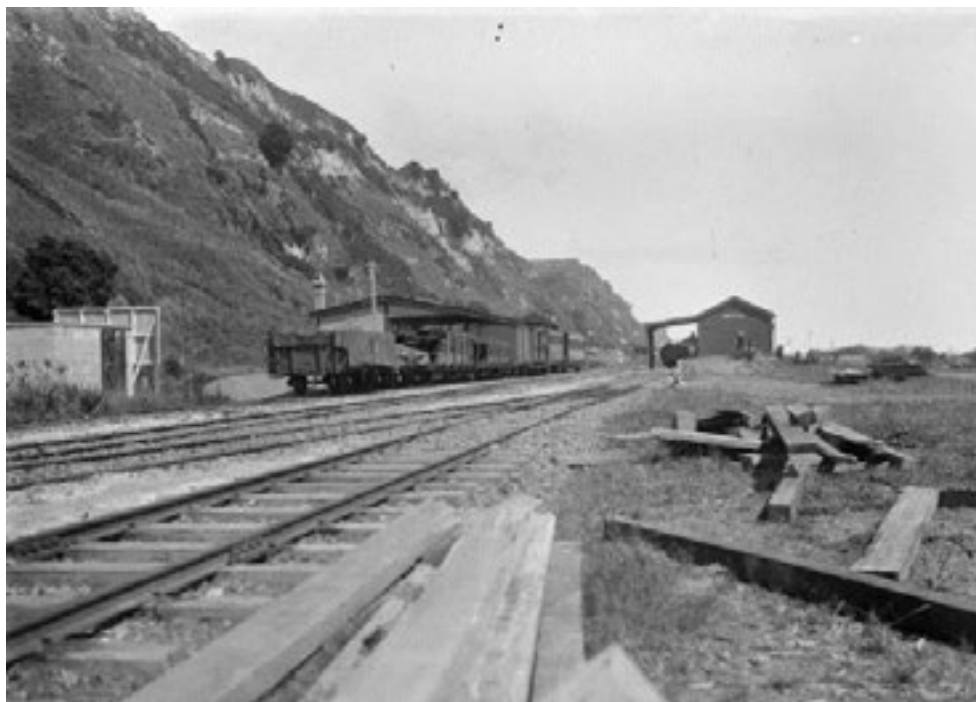
Figure 8.5: View of the former Matatā railway station in 1924. The station was located approximately where the current oversized load bypass rejoins SH2. Note the numerous areas devoid of vegetation and the significant talus slope developed at the base of the escarpment (reproduced with permission of Alexander Turnbull Library)
