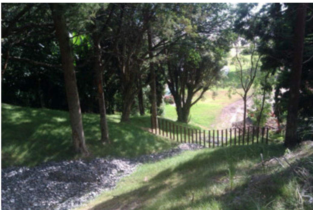
Figure 12.2: Line of steel posts providing protection across a potential landslide path, West End Road, Ōhope
