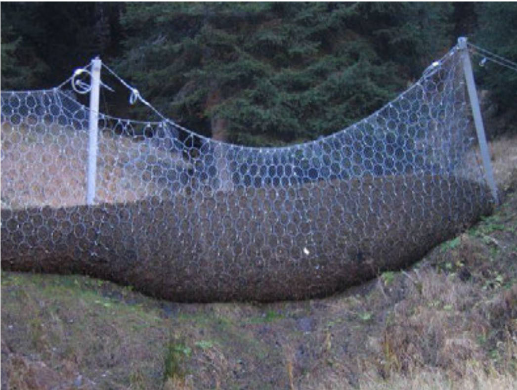
Figure 12.4: Example of flexible ring-net barrier
