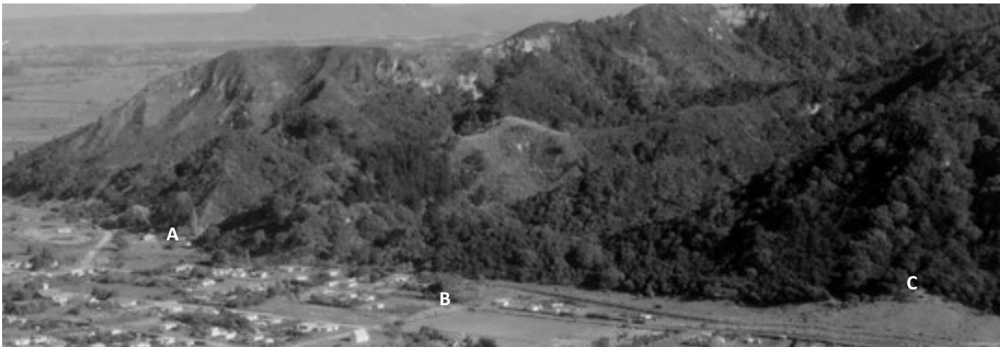
Figure 8.8: View of Eastern & central Matatā in 1965: Waitepuru Stream (A); Division Street (B); Debris Fan (C). Note the limited elevation of the escarpment compared to that west of the town (reproduced with permission of Alexander Turnbull Library)
