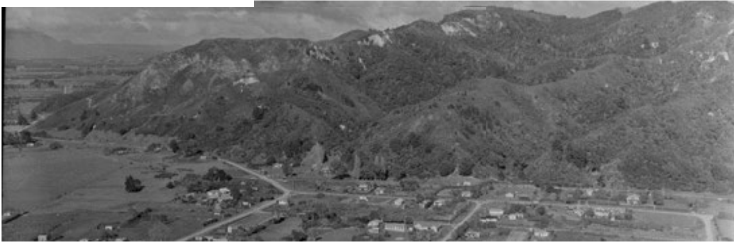
Figure 8.7: View of eastern and central Matatā in 1951 (reproduced with permission of Alexander Turnbull Library)
