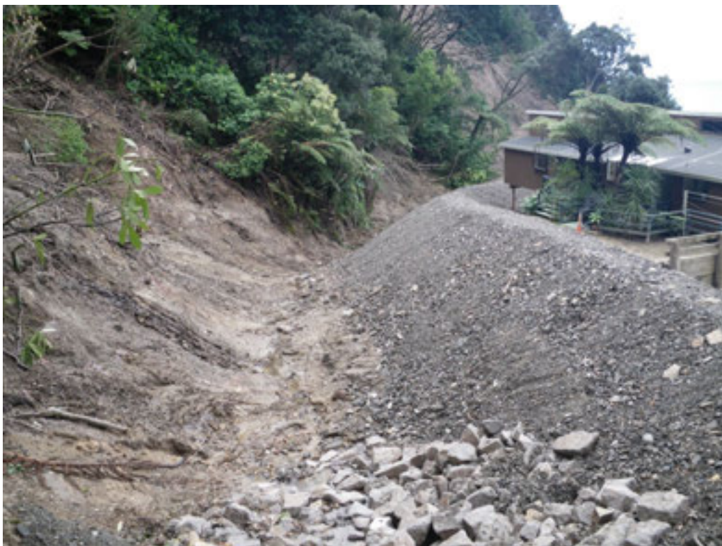
Figure 12.1: Earth bund constructed behind 71/71a West End Road, Ōhope
