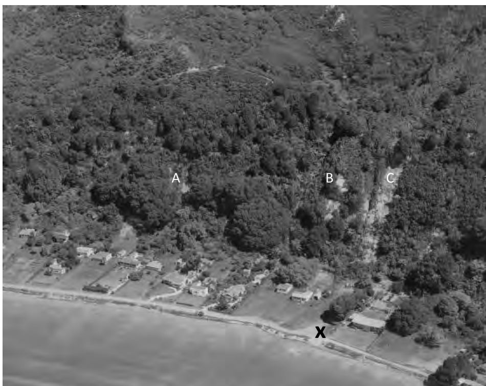
Figure 9.2: West End Road, Ohope, 1955. Slips identified in the text are indicated. "X" indicates the estimated location of where Figure 9.1 was taken. A large pohutukawa effectively blocks much of the Fleming (1955) slide ("A") from view (Reproduced with permission of Alexander Turnbull Library).
