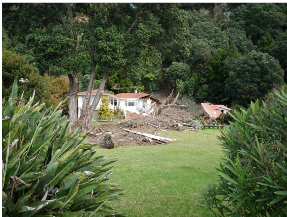
Figure 7.3: View of highly fluidised debris which travelled significantly beyond the recognised extent of the talus slope at 67 West End Road in 2010.
