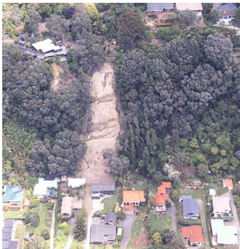
Figure 9.4: View of the large landslide that occurred above below No. 14 Cliff Road in July 2004. The affected properties at the base of the slope are No. 34 and 35 West End Road. Immediately to the right of the landslide scar is the location of the large landslide recorded in Fleming (1955). This section of slope was fully vegetated by 2004.
