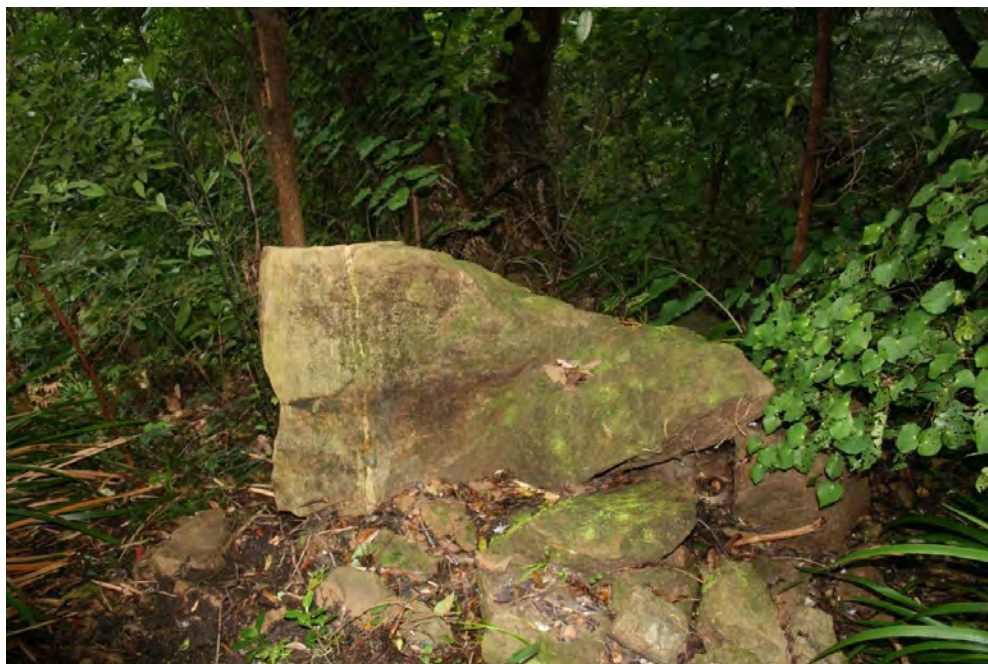
Figure 9.7: Sandstone boulder and smaller rock debris on the talus slope behind the West End property where a rockfall fatality is reported to have occurred in 1959.
