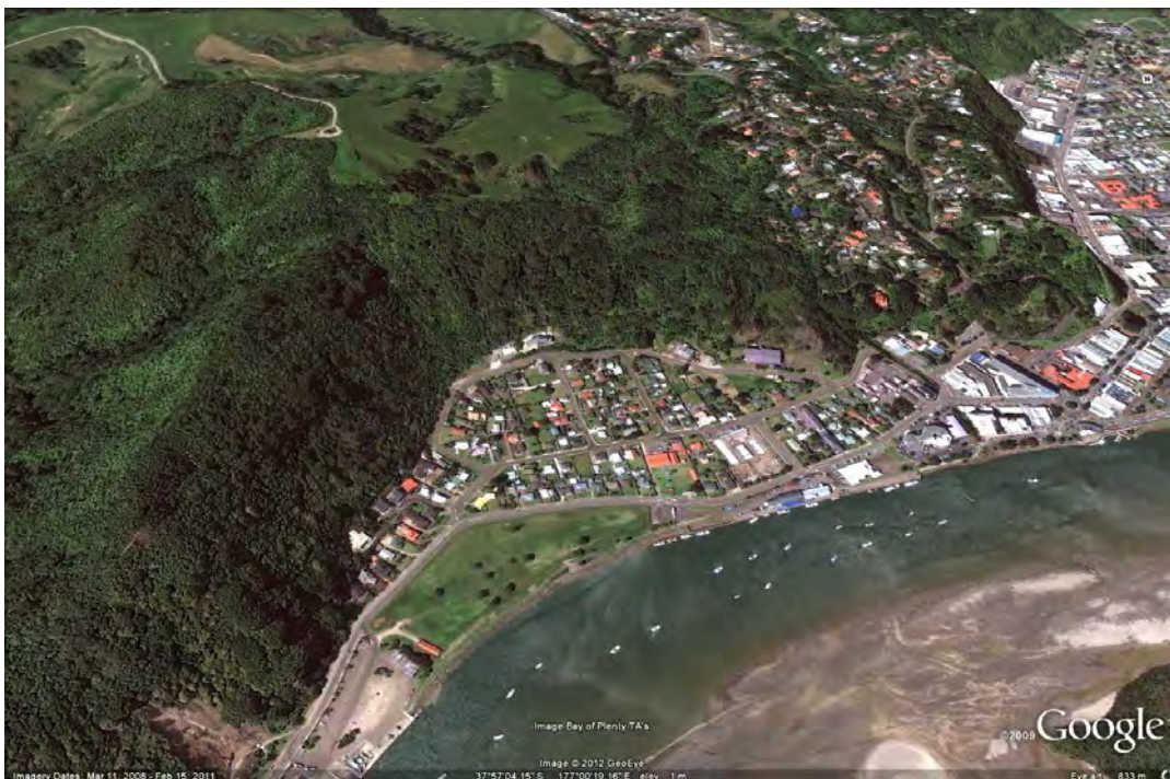
Figure 8.2: Google Earth oblique view of the Wepiha St/Harvey St area showing a near complete vegetation cover (aerial photo dated February 2011).
