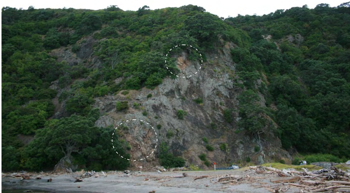
Figure 8.9: Minor rock falls within highly jointed greywacke (circled), Whakatane Heads.
