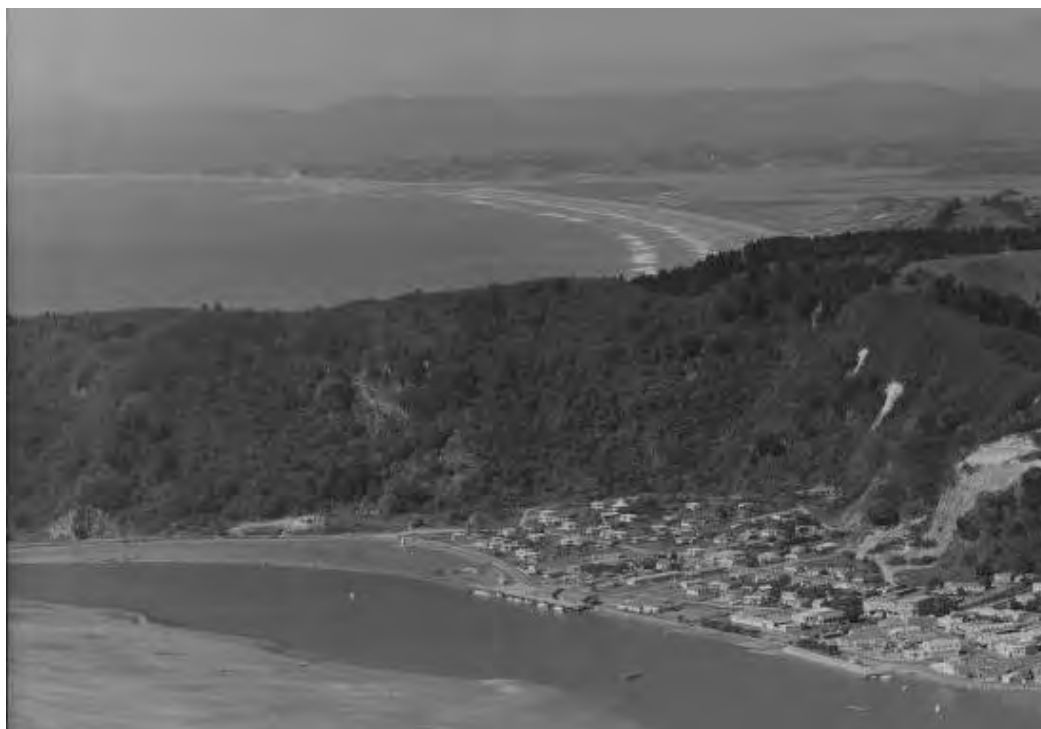
Figure 8.3: View of the Wepiha/Harvey Street area in 1964. Two apparently recent landslides within the Ohope Beds can be seen on the right (Reproduced with permission of Alexander Turnbull Library).
