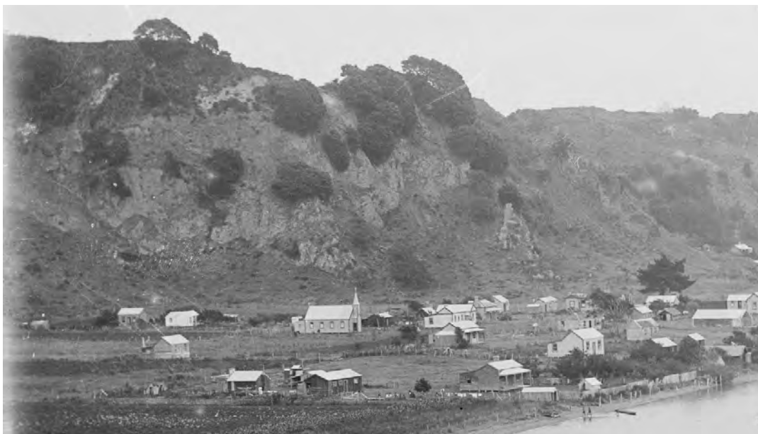
Figure 8.1: View of the Wepiha St/Harvey St area c1900-1910 showing the presence of shallow landslides within the Ohope Beds. A talus slope has developed below the denuded greywacke rock face (Reproduced with permission of Alexander Turnbull Library).
