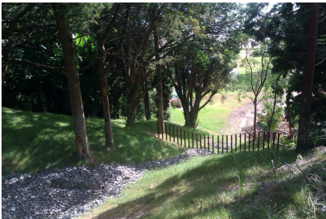
Figure 16.2: Line of steel posts providing protection across a potential landslide path
