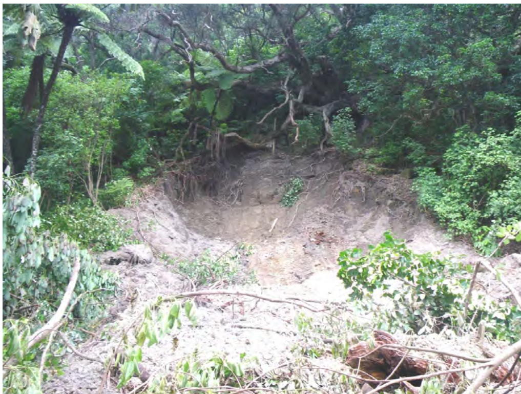
Figure 9.6: Landslide within the talus slope behind West End Road. A large pohutukawa tree mobilised by the landslide caused sufficient damage to the adjacent dwelling.
