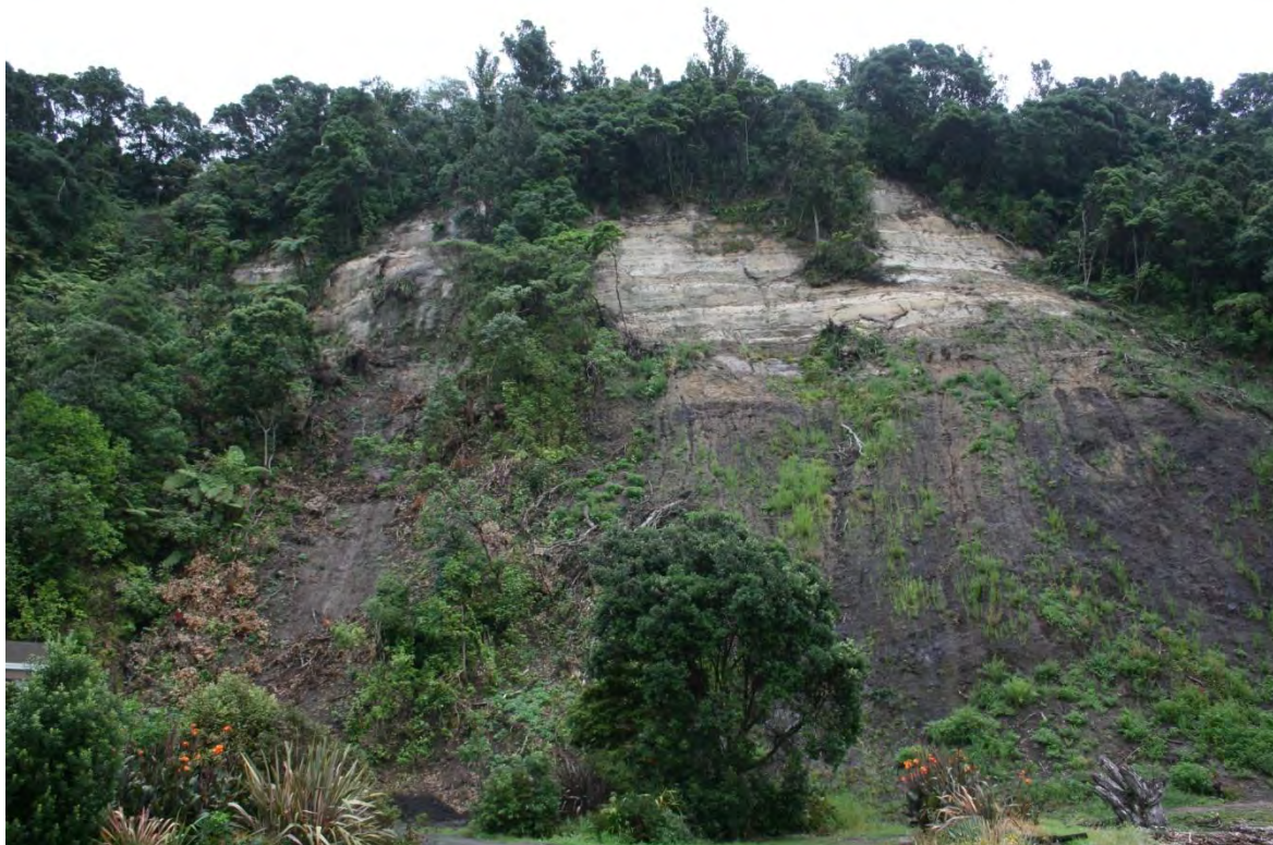
Figure 9.12: Shallow failure of the very thin soil and vegetation cover from a steep face formed from the Lower Ohope Beds. The debris also removed the vegetation cover of the underlying greywacke.
