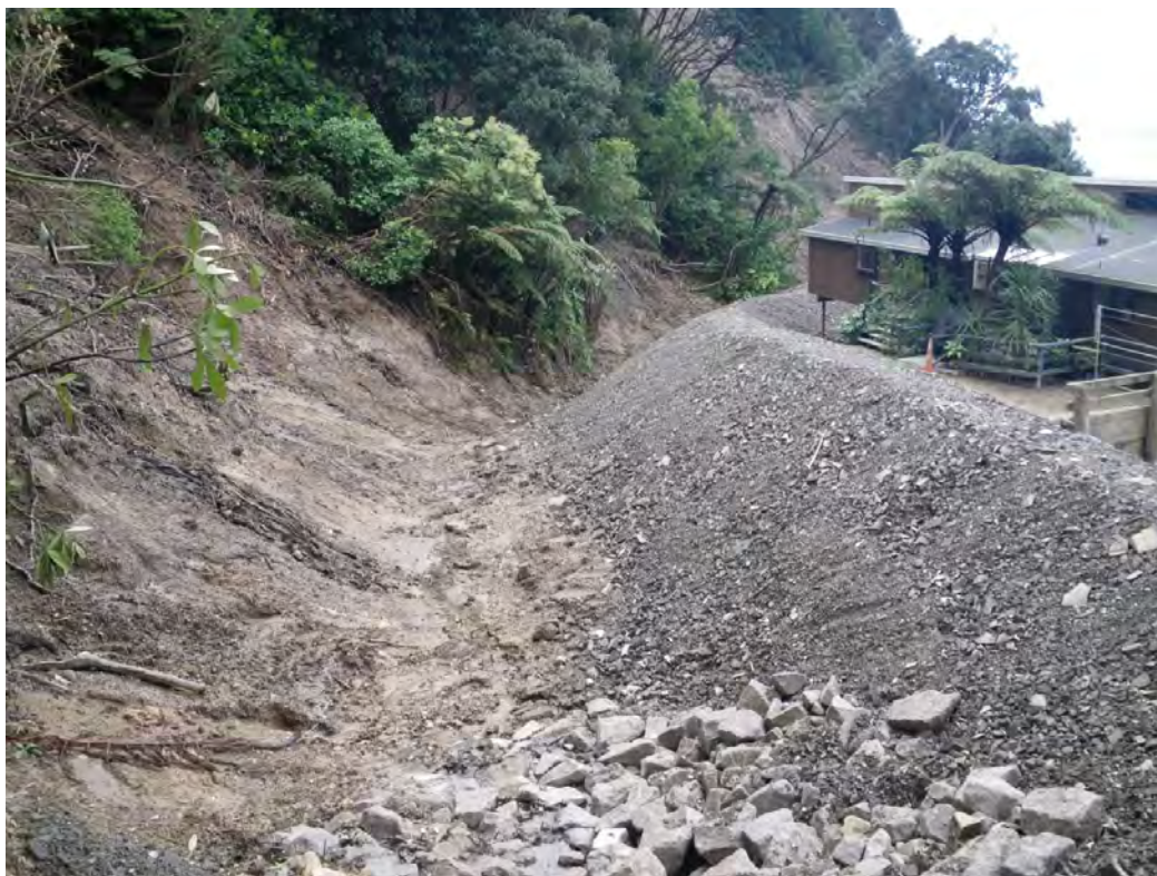
Figure 16.1: Earth bund constructed behind 71/71a West End Road
