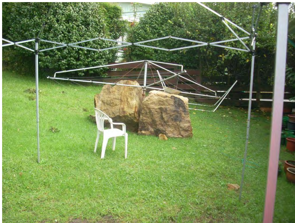
Figure 9.9: Rock fall at the rear of a property on Pohutukawa Ave, Ohope.
