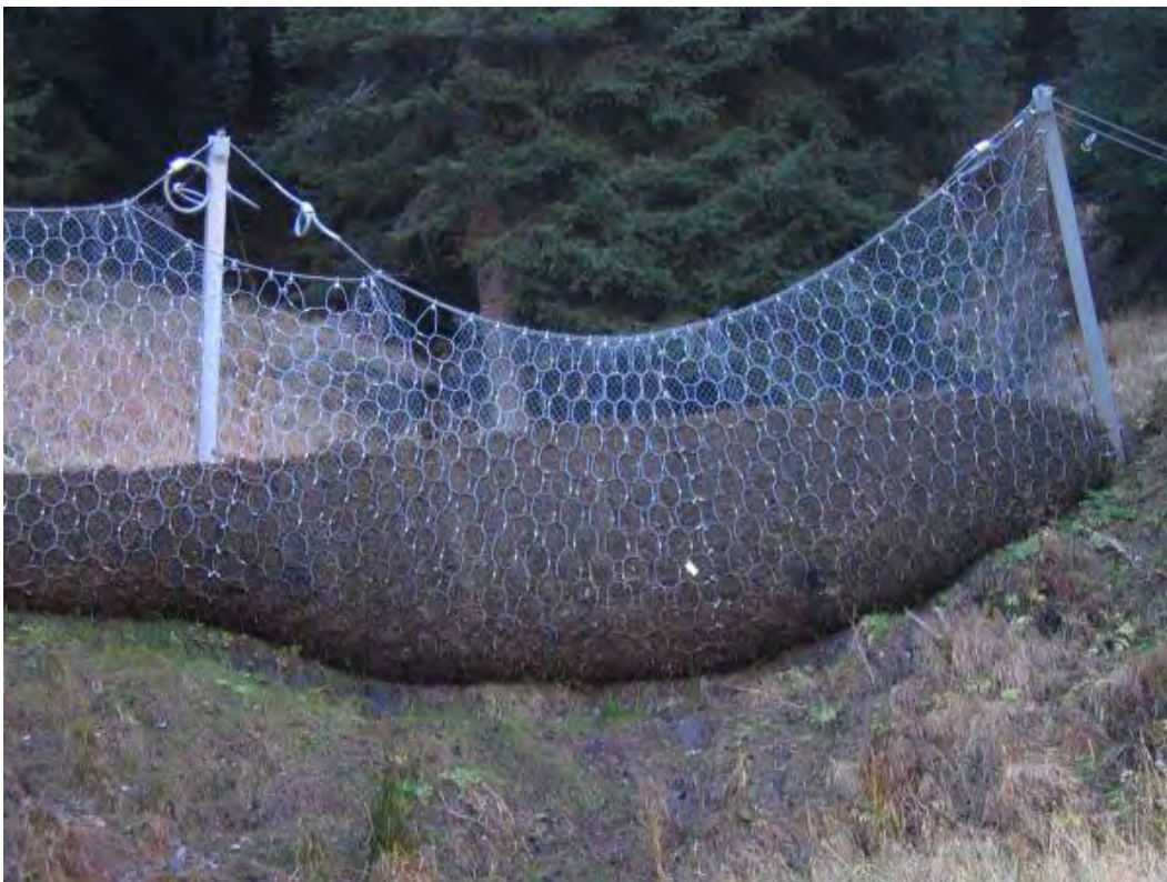
Figure 16.4: Example of flexible ring-net barrier
