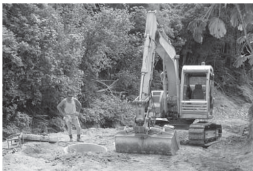
Hazard Mitigation Works at Otarawairere
