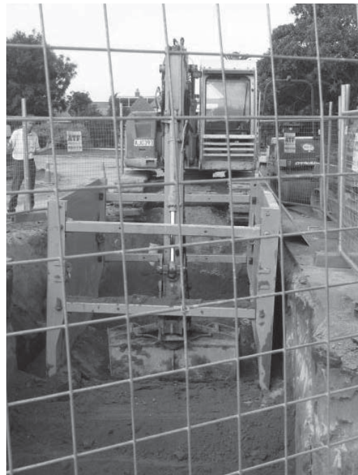
Works at Otawairere
