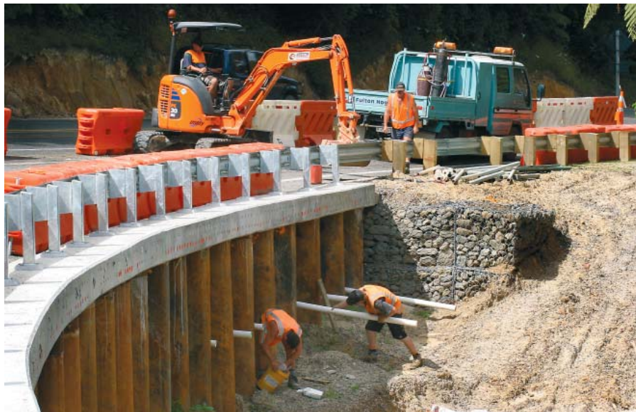
Ohope road rehabilitation programme.
