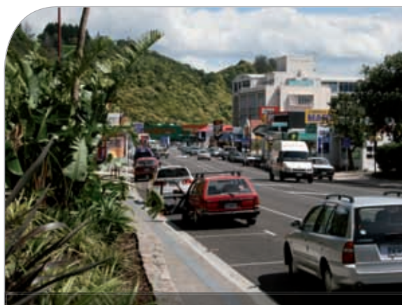
View from the northern end of Commerce Street following completion of the upgrade.
