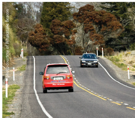
Ohope Hill Road safety upgrade
