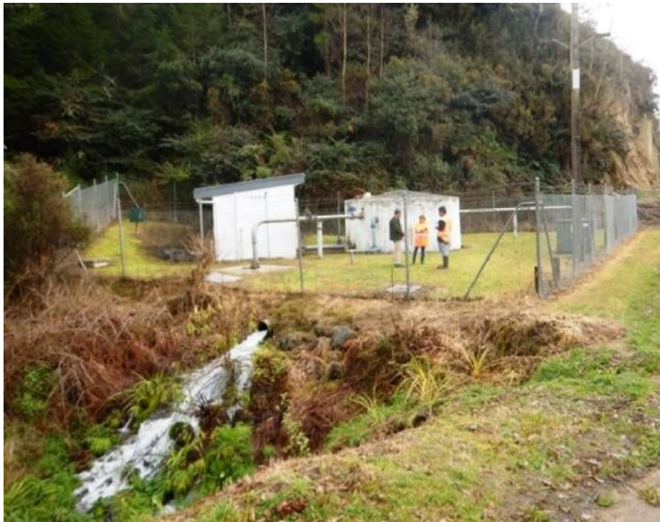
Figure 4: Pump Station Site with Bores and Suction Tank (Left) and North Bore Head (Right)
