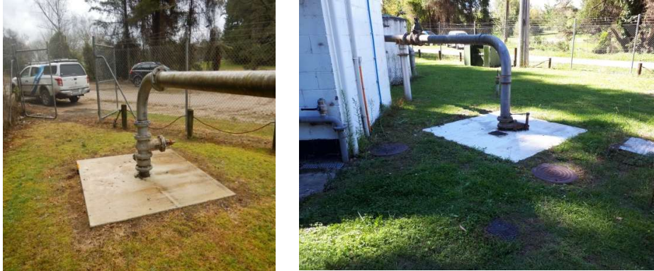
Figure 5: North Bore Head (Left) and South Bore Head (Right)
