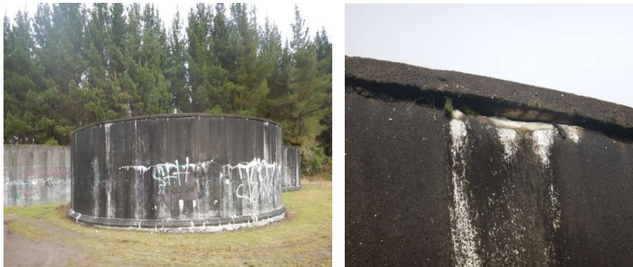
Figure 7: Concrete Reservoirs (Left) and Reservoir Roof (Right)
