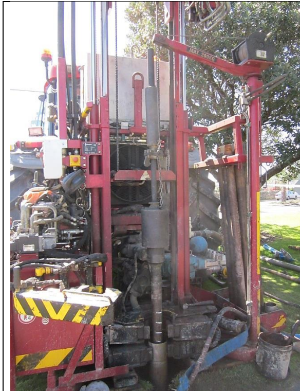
Figure 6. SPT hammer in progress
