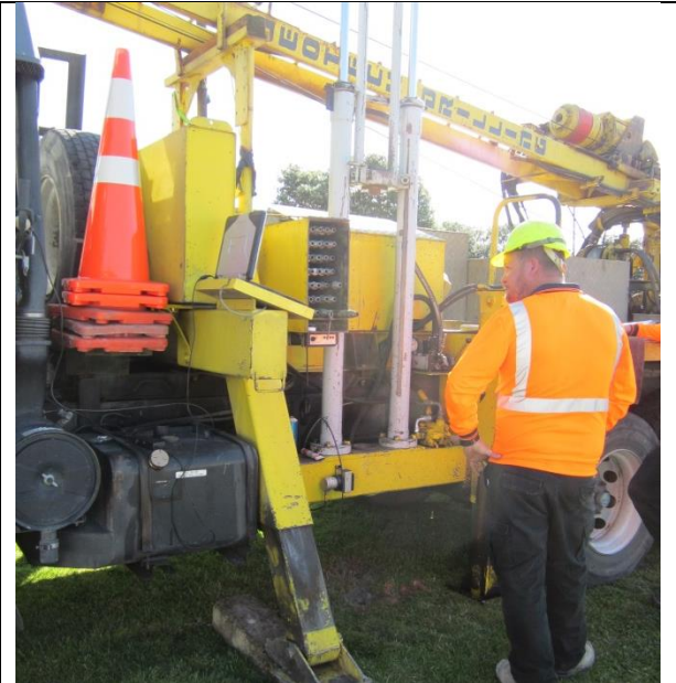
Figure 18. GEOTECH CPT rig, zero'ing electrics
