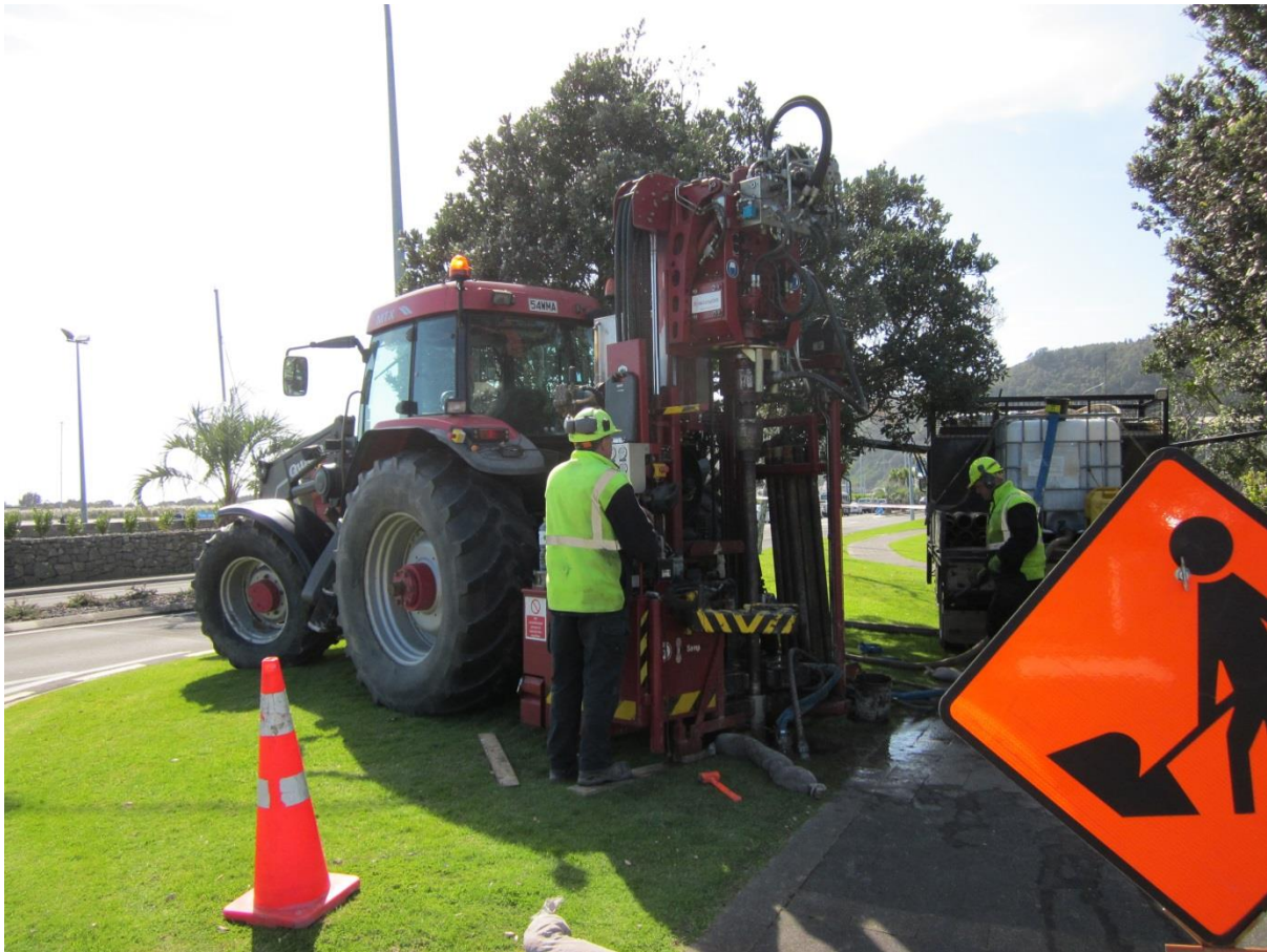
Figure 1. GEOTECH sonic rig, BH 4
