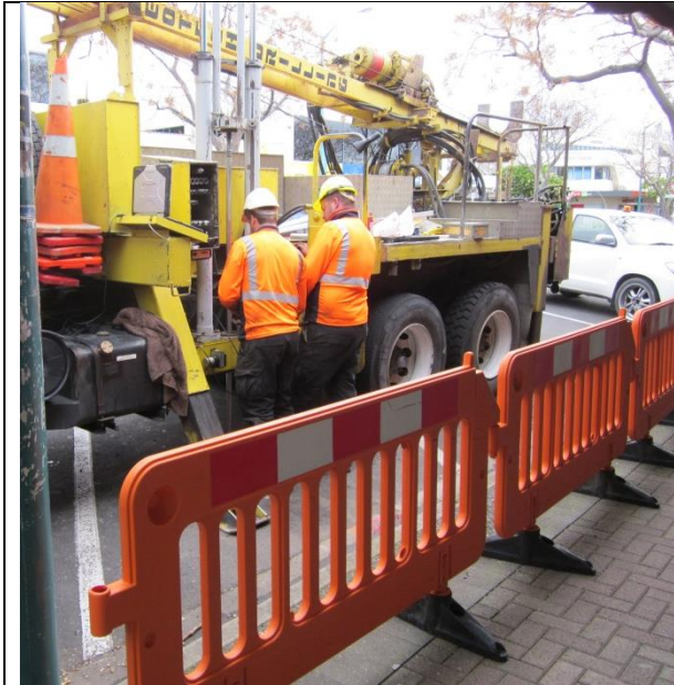
Figure 17. GEOTECH CPT rig on Strand, note pedestrian management
