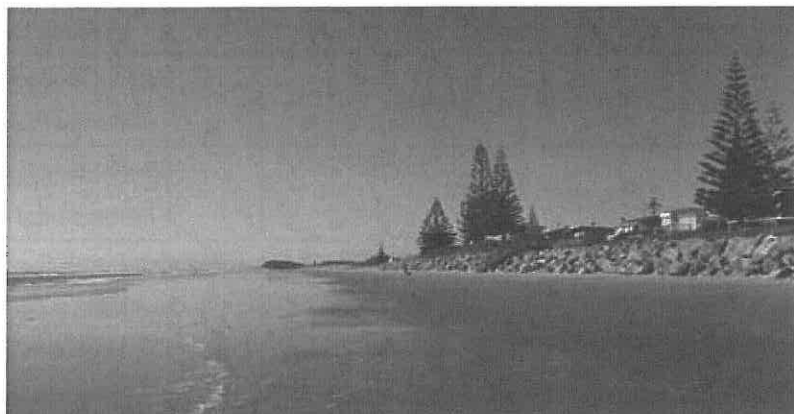
Coastal Protection works, Waiti Beach
