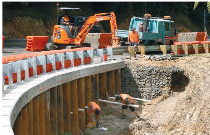
Ohope Road rehabilitation project.
