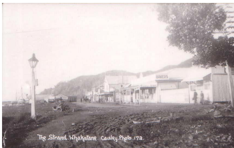
View along The Strand prior to reclamation. WMG no P1145
