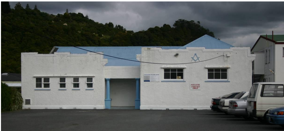
Masonic Lodge Building
