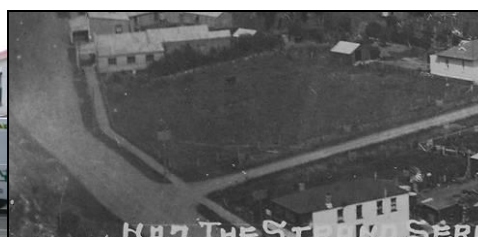
The corner site prior to construction of Shapley's. No date
