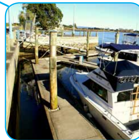
Quay St Wharf Extension
