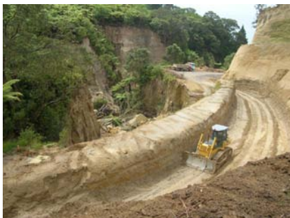
Herepuru Road under construction
