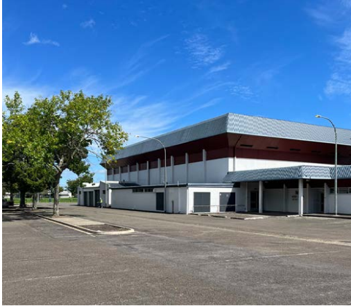
REAR OF WWMH - SOUTH
