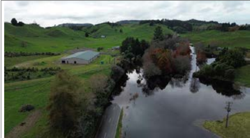
Drone photo of flooding looking east – May 2023
