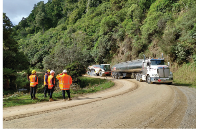
Inspection of tall oil pitch application
