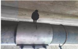
Council received advice from a kayaker that there was a leak in the water pipe under the bridge. Investigation showed the leak was on an elbow of an air valve fitting. An air valve is necessary in this location as it is the highest elevation of the pipe. Air release is necessary to prevent flow restriction. The concrete lined galvanised spiral welded steel pipe has an internal diameter of 210 mm and is the sole supply to all consumers on the western side of the bridge.
