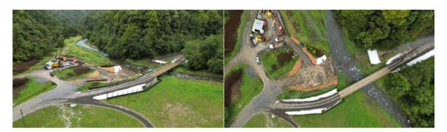
Piling has been completed on the western abutment. This was a high-risk activity in relation to the programme and so was a major milestone to achieve. Riprap levels have now been confirmed and excavation will start once ground water levels are reduced. In the coming weeks we will see riprap installed on the Eastern end, sheet piles installed around the central pier and concrete works to get the bridge out of the ground at both locations.
