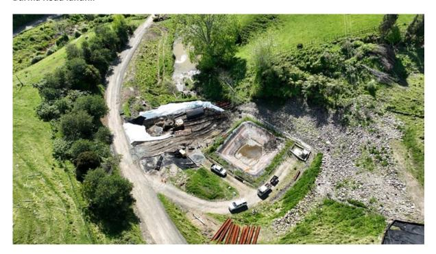
Work on the site is progressing well, with the leachate collector chamber now substantially complete. This chamber is designed to capture and collect leachate—the liquid that drains or 'leaches' from a landfill or waste storage area. Installation of the new leachate collector drains, which are part of the landfill's drainage system to channel leachate into the chamber, is also underway.
