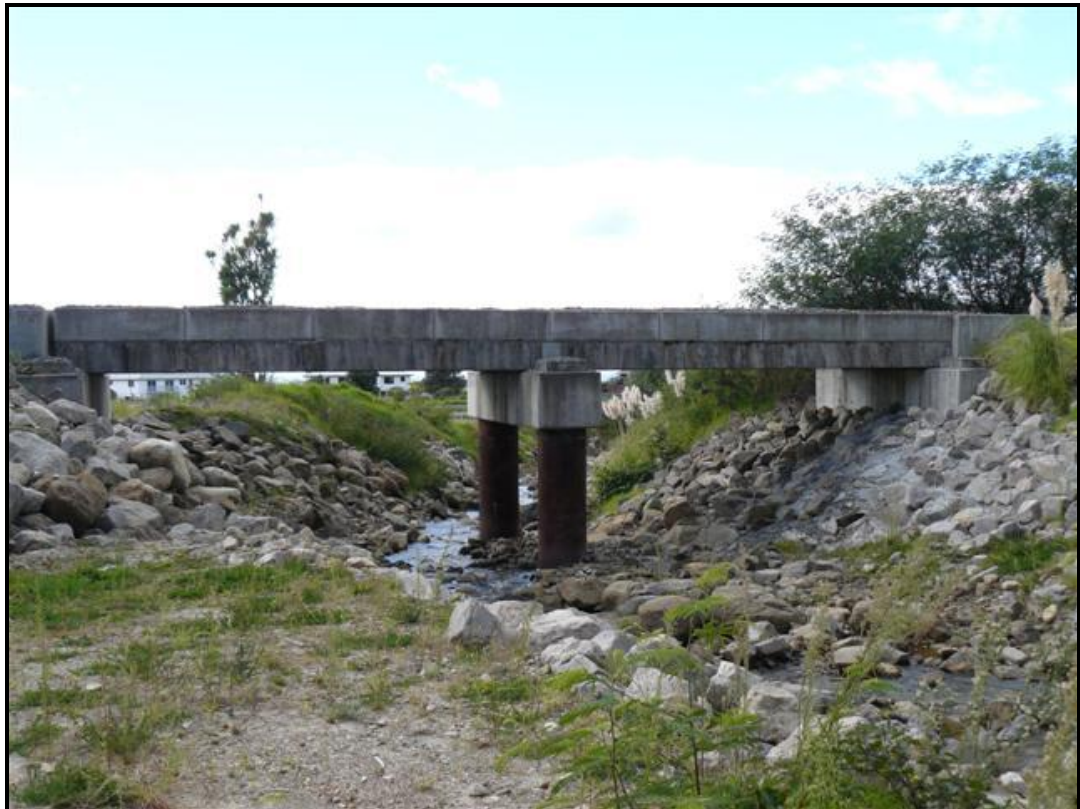
TWIN SPAN ECMT RAILWAY BRIDGE (Note central pier)
