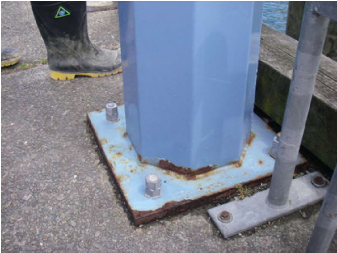
Photo T13 - pole on wharf (1940 section)
