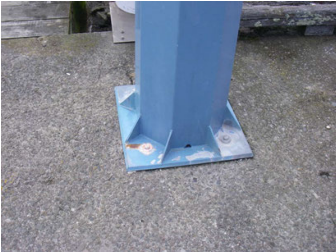
Photo T02 - pole at east end of wharf
