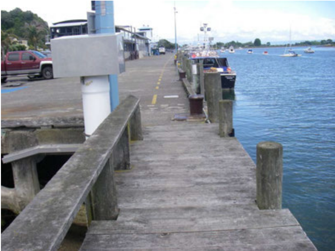
Photo T01 - view from east end of wharf
