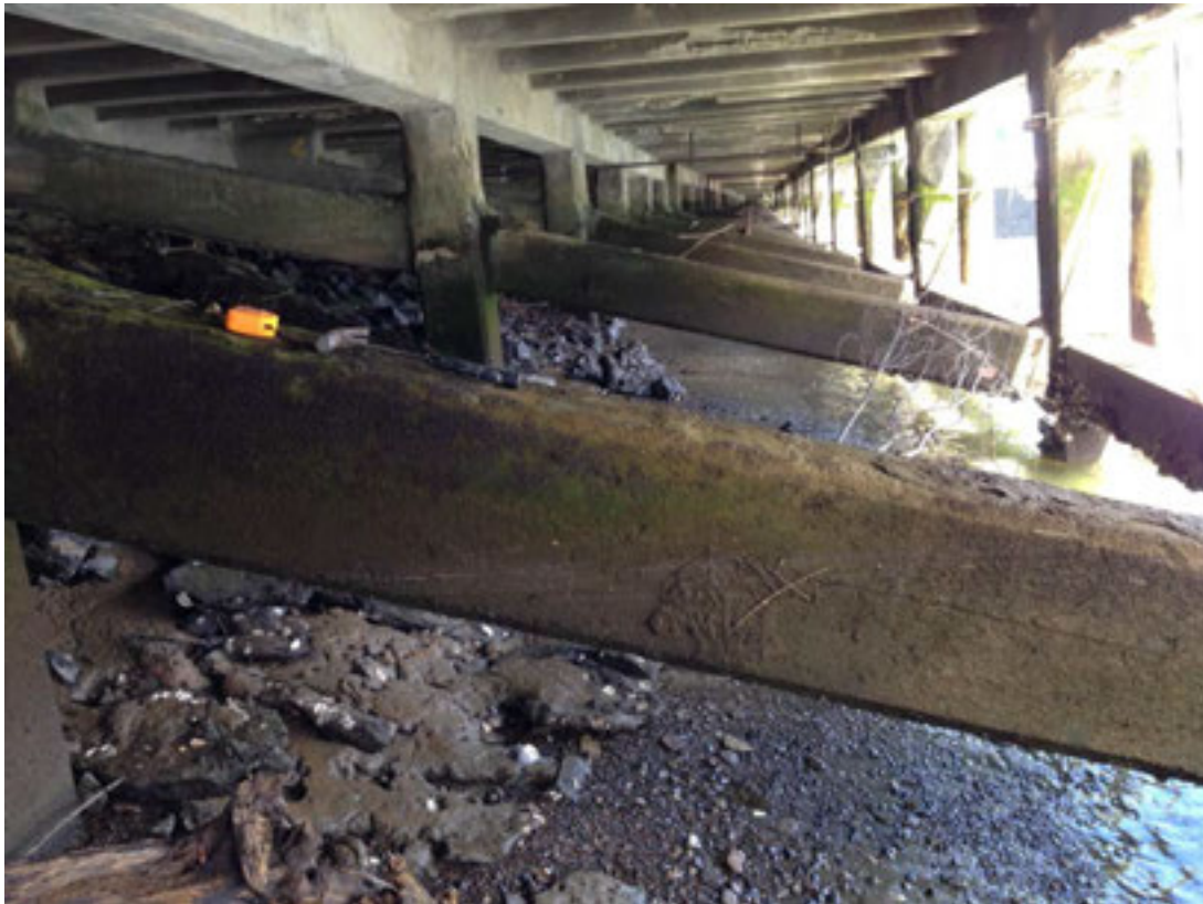
Photo A09 - View along wharf from gridline A2
