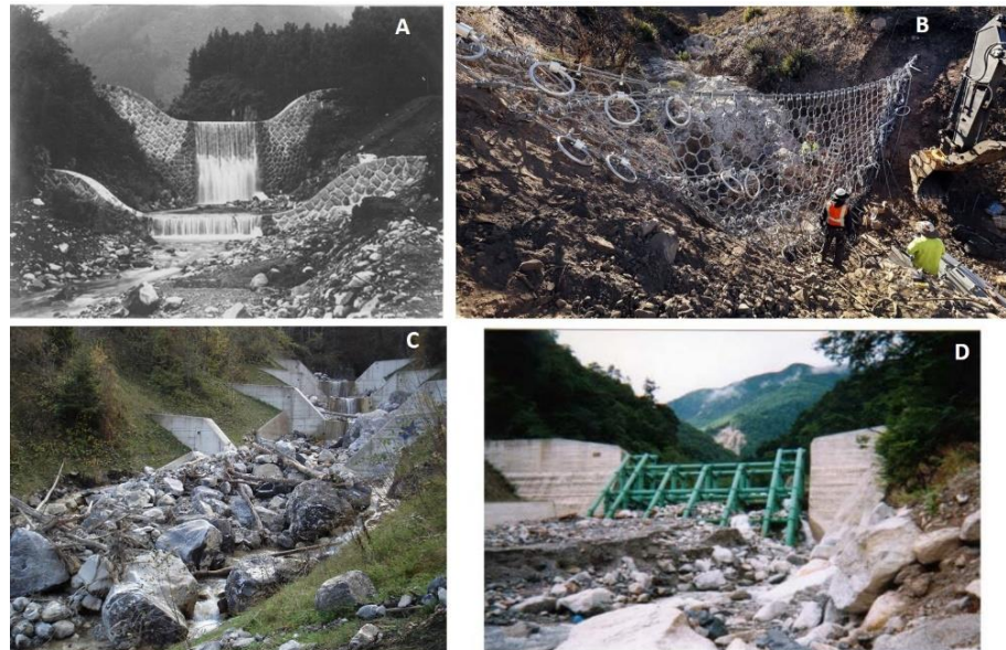
Fig. 3 Examples of debris-flow structures. A: Masonry dam. B: Ring-net. C: Check-dams. D: Grill.
