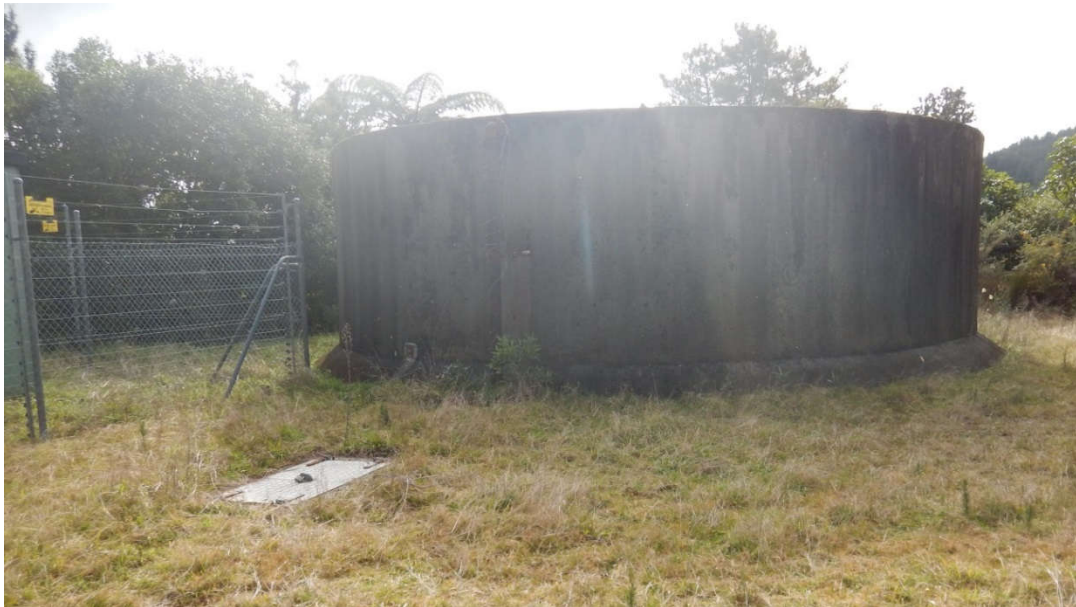
Figure 8: Concrete Storage Reservoir
