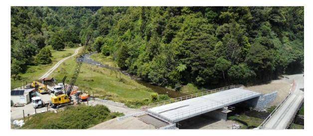
Work continues and nears completion for the Mimiha Bridge replacement. The bridge beams have been set, bridge abutments and earth stabilised. Retaining walls continue to be constructed and the bulk fill for the approaches has started.
